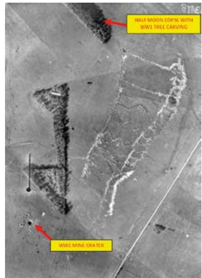
Fig 13 - Bustard trench system and mine crater. 1920 Aerial photograph. It is not clear where the entrance was for the horizontal passage (adit) dug by the miners to plant the mine.
